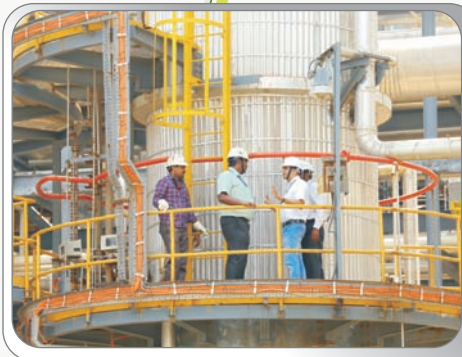
CT Type Inspection at CDU III DA31006 NDT Test
